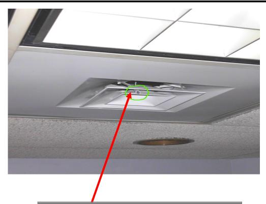
Male cable connector can be located at the diffuser discharge eliminating the need for the Ceiling Receptacle. The male connector can be held securely in place and out of sight by a "peel-and-stick" plastic clip that is also available through Arrow United.
