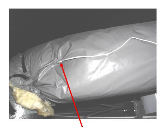
Plenum rated cable can be routed along the outside of the flexible ductwork and then cut into ductwork just above the plenum discharge.
