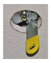
At right is shown the optional **Ceiling Receptacle bracket finger** after the hard ceiling panels have been installed. This is what the balancing technician sees at each damper location.
